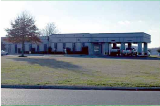
Two drive-thru lanes were added to the Chase Customer Service Center to better assist customers.
